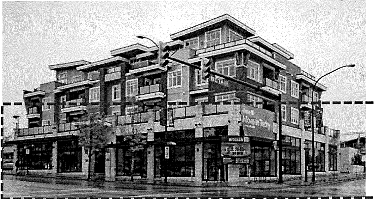
The three commercial/retail and office strata units are outlined in the blue dash line.
